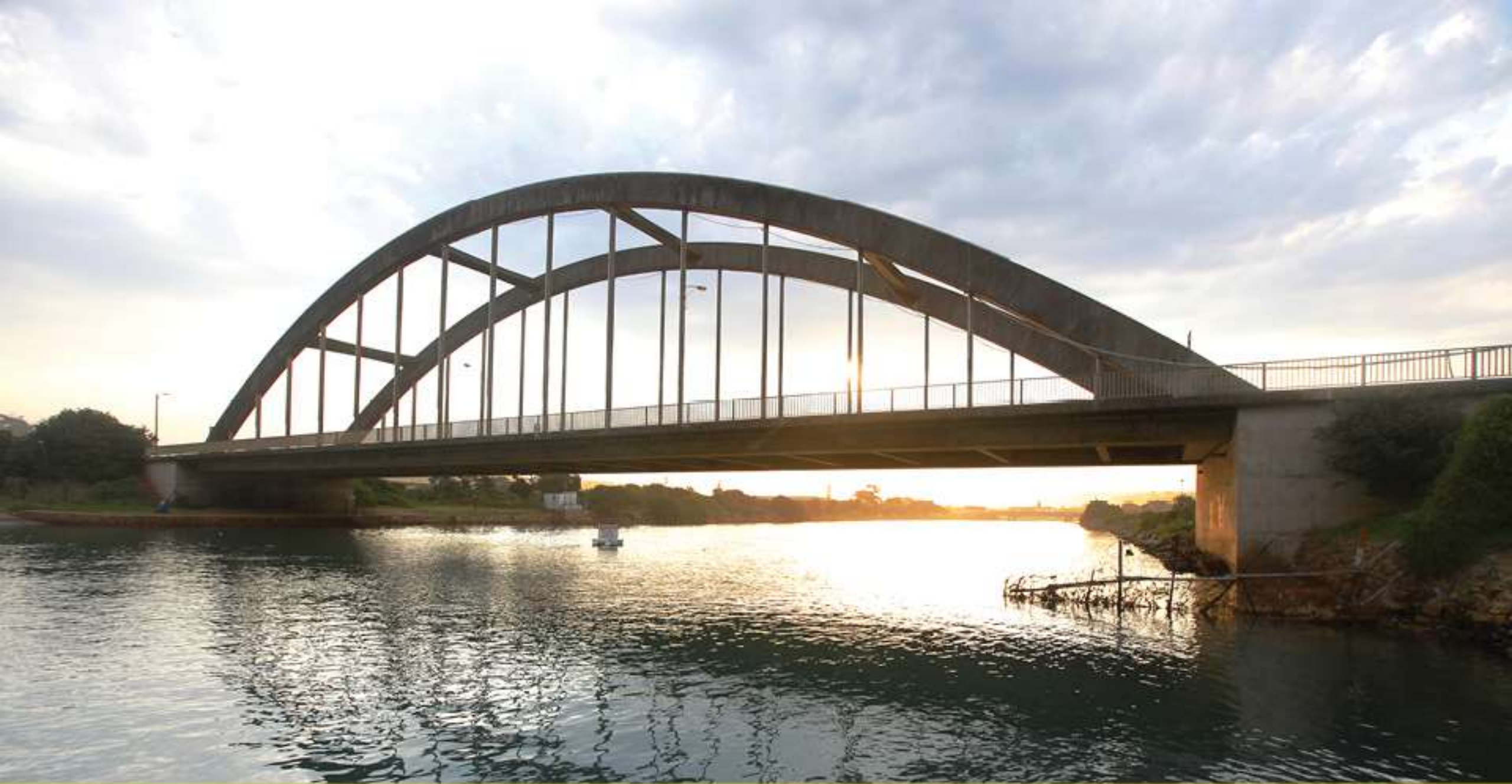
Port Alfred Bridge
